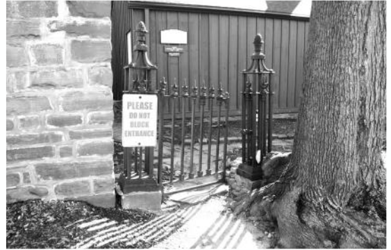
This old iron entrance at the Society's offices, 110 King St. has seen better days. One post has been enveloped by a tree, whose roots are spreading onto the path, making it difficult for visitors to safely enter the narrow opening. The Coach House is to the left.
