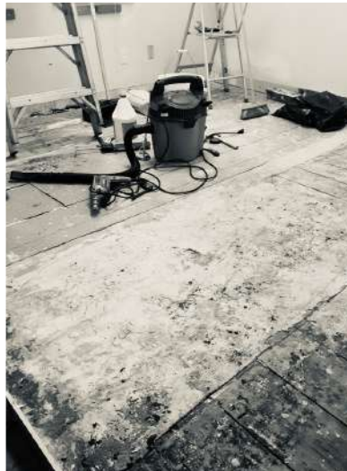
Archives Room - Before
