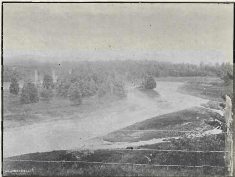
DAM AND RAILROAD BRIDGE—LOOKING WEST.
