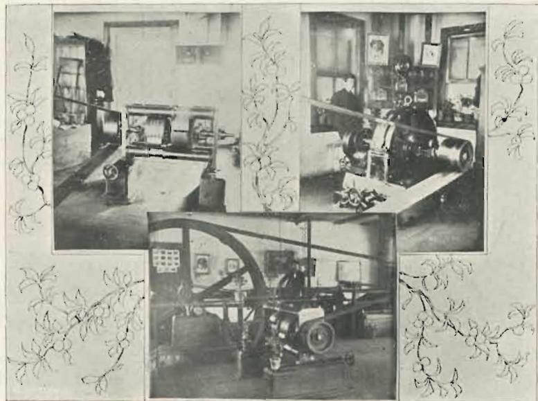
INTERIOR ELECTRIC LIGHT PLANT, R. MCGOWAN, PROP.
