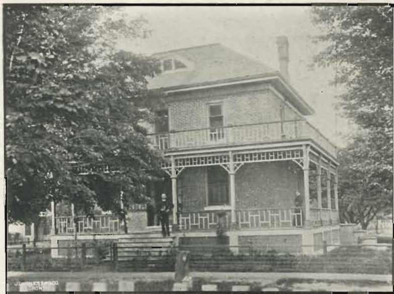
ST. ANDREW'S PRESBYTERY, RESIDENCE OF REV. R. T. BURKE.
